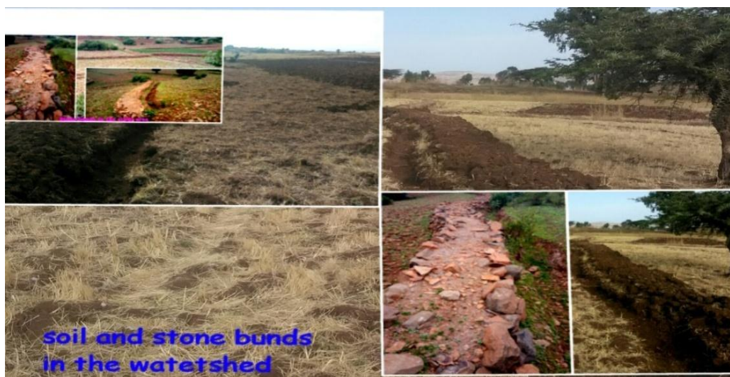
Figure 4.2. Soil and Stone bunds which are constructed by the community in the study area
