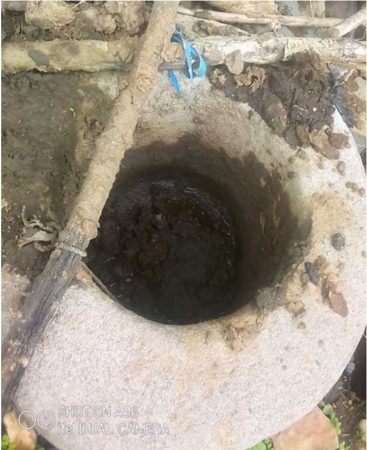
Figure 4: Dung stored in the inlet pit for later use
