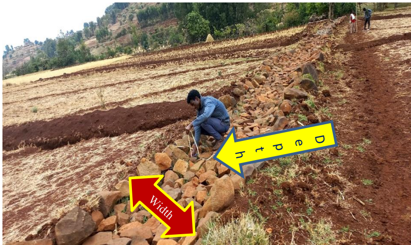
Figure 4.1 Measured waterway from study area (field survey, 2022)
