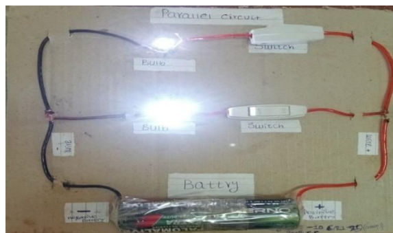
The switches are on
