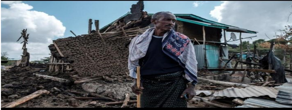
Figure 2.3. An example of a damaged house in NWE livelihood zone (Kobo town Communication Office, 2023)
