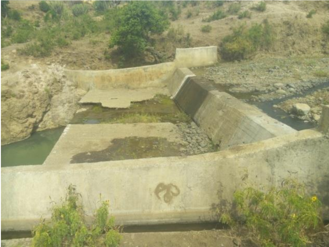
Figure 3-2 Amiba Garno irrigation headwork structure
