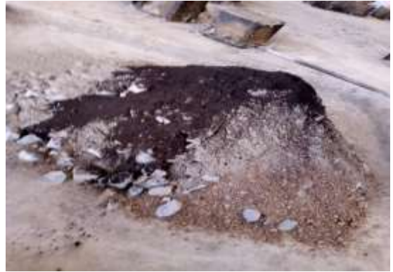
Batching of concrete
