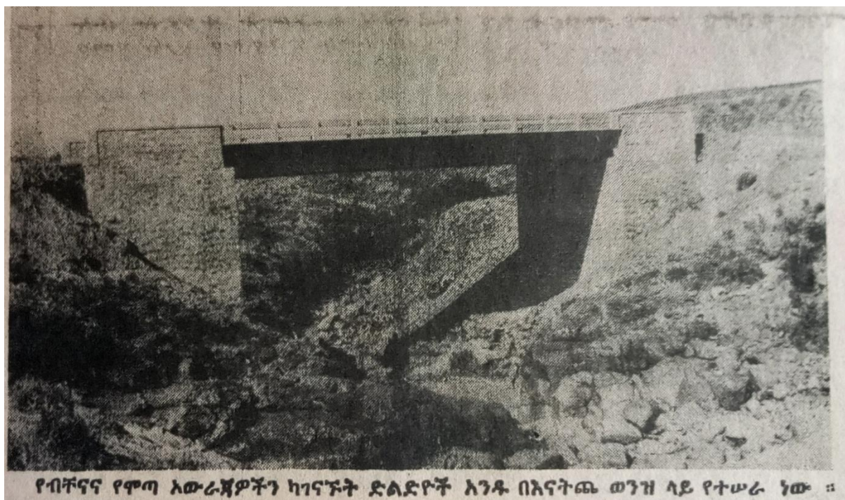
Figure 40: A concrete bridge built on the Inat Çä River along Däjän to Moṭṭa feeder. Source: Addis Zemen Newspaper, Sene-Nehase (June-August) 1970 E.C.
