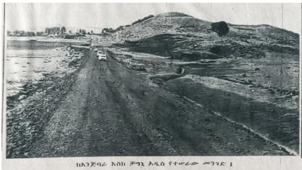
Figure 38: A new road constructed from Injibara to Čagni. Source: Addis Zemen Newspaper, Hamile-Pagumé (July-Pagume) 1971 E.C.
