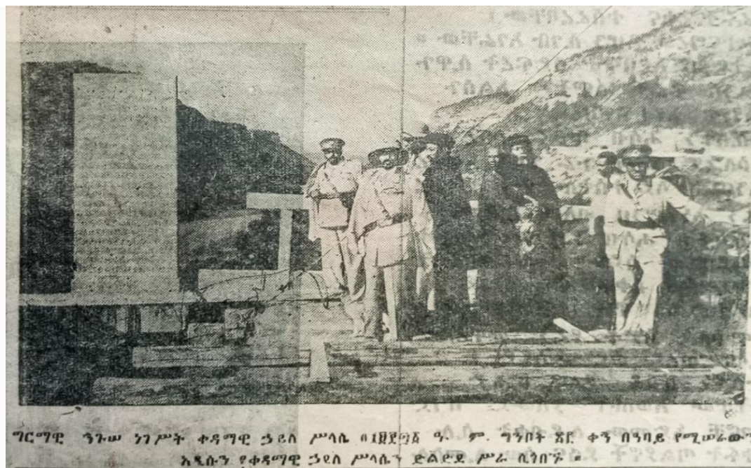
Figure 29: Emperor Haile Selassie Accompanied by Abune Basilios visiting the construction of the Blue Nile Bridge. Source: Addis Zemen Newspaper 9 th year, 1941-1942.
