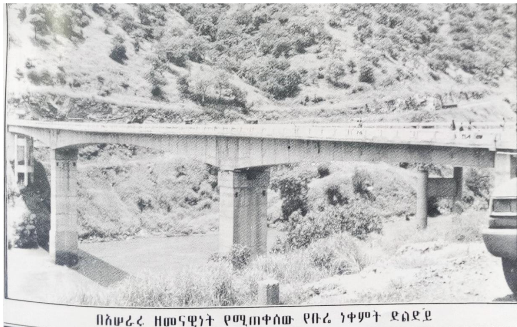
Figure 41: The modern concrete bridge built on the Blue Nile River along Buré-Nāqämit road. Source: Ethiopian Roads Authority Golden Jubilee, p.51.
