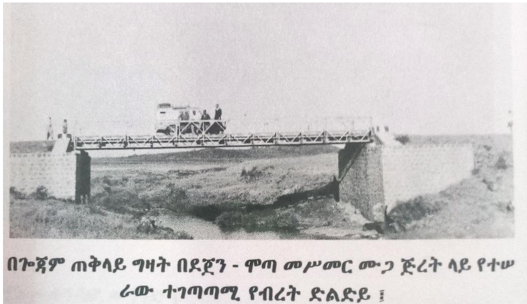
Figure 42: Bailey bridge built on the Muga River along Däjän-Moṭṭa feeder road. Source: Eighteenth annual report of the Ethiopian Road Authority, P.2.
