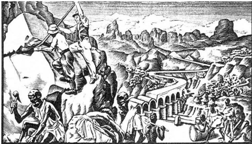
Figure 8: Labor based highway construction by Italians. Source: Antonsich, “Sign of power: fascist urban iconographies in Ethiopia (1930s-1940s)...,” p. 333.
