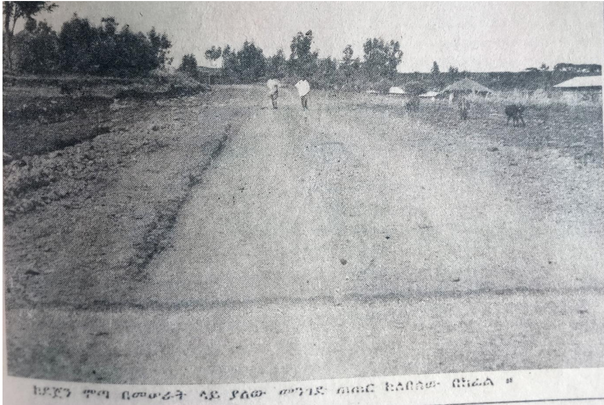
Figure 38: Partial view of the road from Däjän to Moṭṭa under construction. Source: Addis Zemen Newspaper, Hamile-Nehase (July-August) 1968 E.C.
