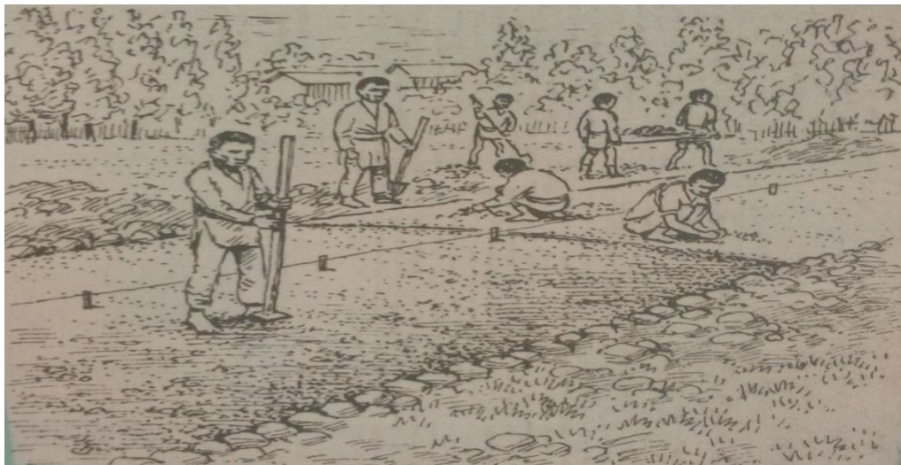
Figure 3: Addis Ababa-Addis Alām road under construction. Source: Geoffry Last and Pankhurst, a History of Ethiopia in Pictures , p. 44.
