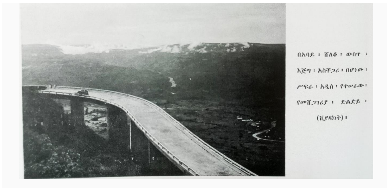
Figure 18: the newly constructed the Blue Nile gorge viaduct. Source: Reports of the IHA, October 1964, p. 24.
