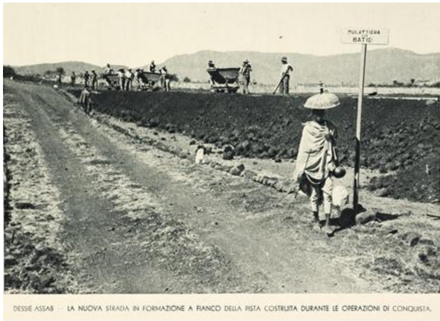
Figure 7: Assäb-Dässé highway under construction. Source: Andrew Denning, “Infrastructural Propaganda: the Visual Culture of Colonial Roads and the Domestication of Nature in Italian East Africa....,” P. 365.
