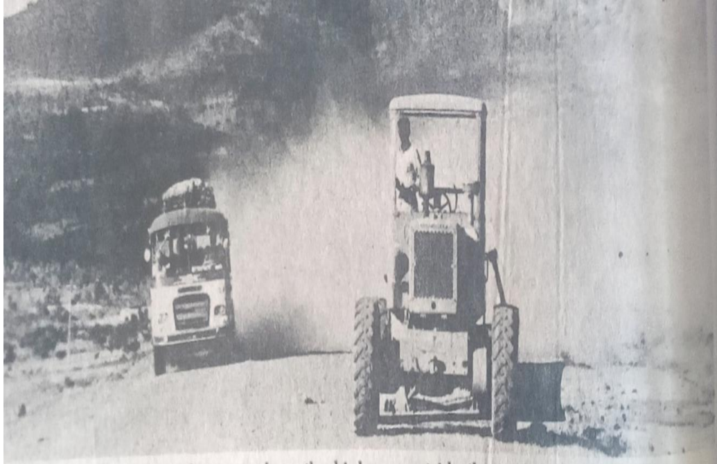
Figure 44: The road grader at repairing work on Däjän-Bahir Dar highway near Injibara. Source: Ethiopian Herald, June-September 1979.
