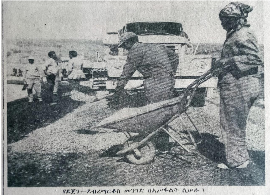
Figure 42: Labor intensive Dājān-Marqos asphaltting work. Source: Addis Zemen Newspaper, Ginbot (May) 1971 E.C.
