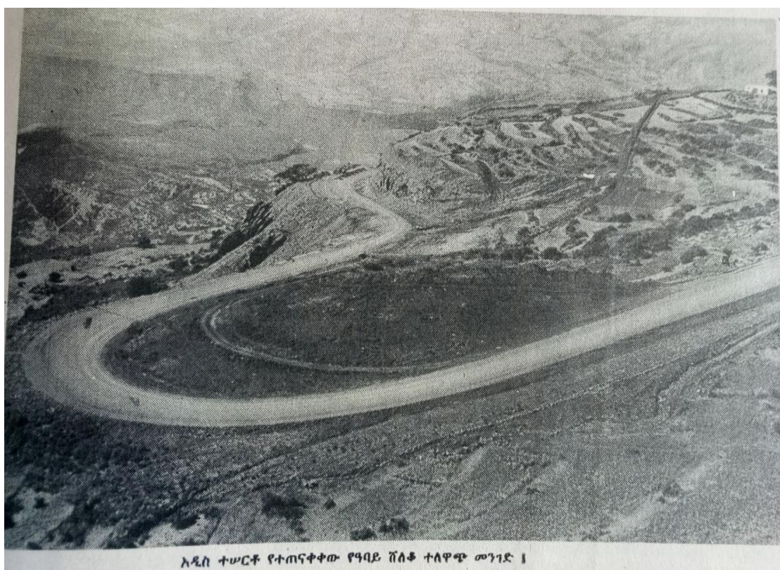
Figure 23: The newly constructed detour in the Blue Nile gorge on the Addis Ababa-Gojjam highway. Source: Addis Zemen newspaper, Hidar-Tahisas (November-December) 1972 E.C.
