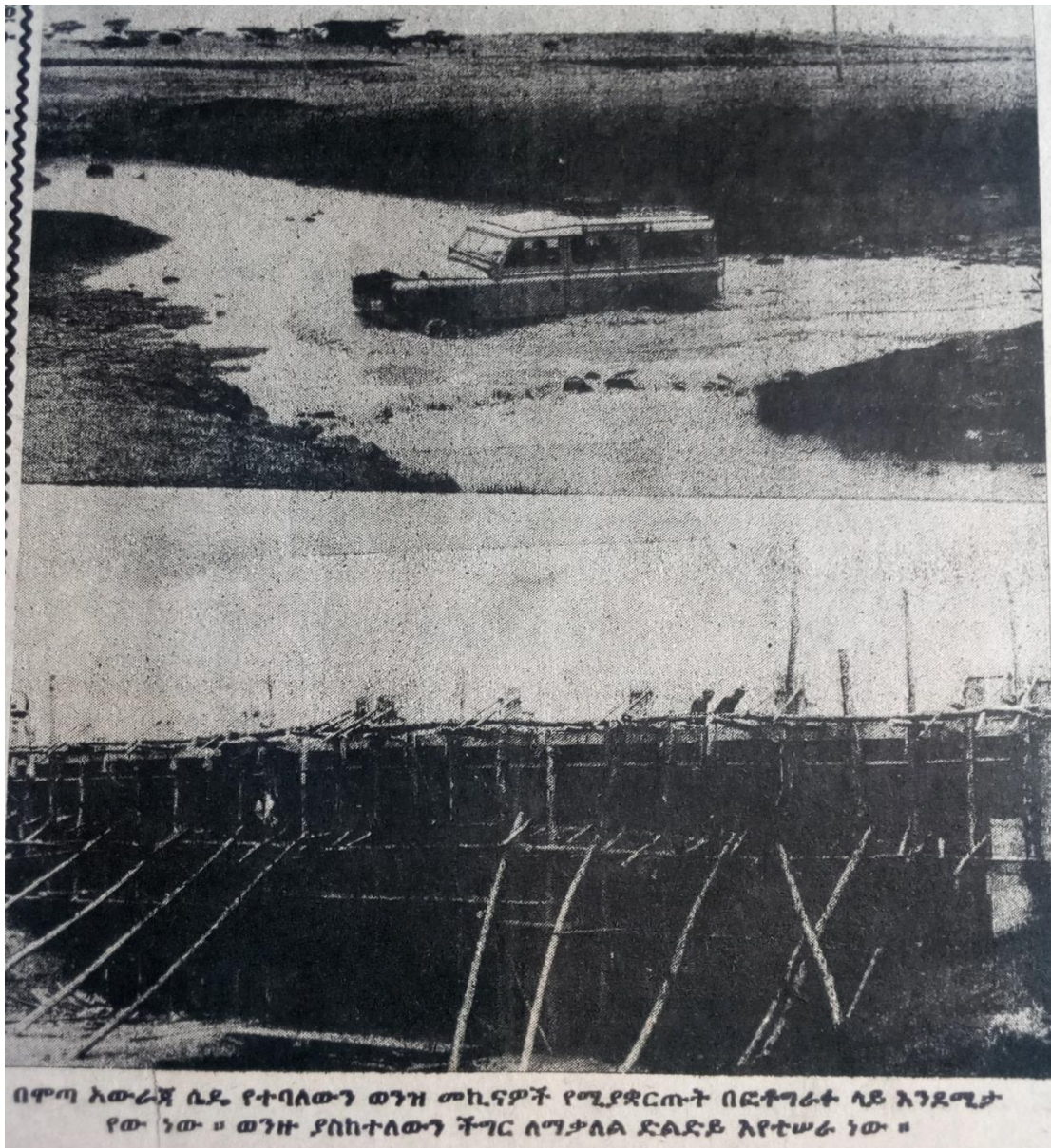
Figure 39: challenges of crossing the river Sädé. To alleviate the challenge, the bridge was under construction. Source: Addis Zemen Newspaper, Yekatit-Ginbot (February-May) 1970 E.C.
