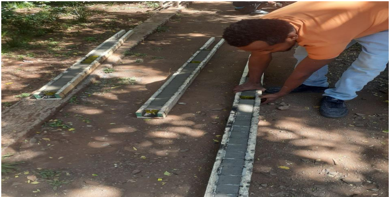
Figure F.5 Some Photo during Work
