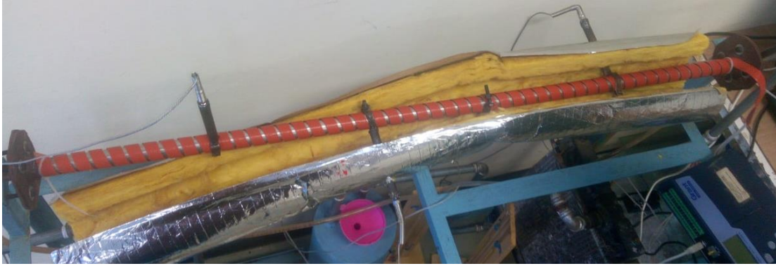
Figure 3-7 Heater tape wrapped around the stainless-steel tube
