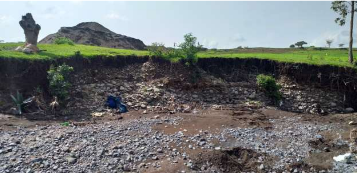
Figure 16(c) (June 07/2019, near Megech main bridge to east direction (left side))
