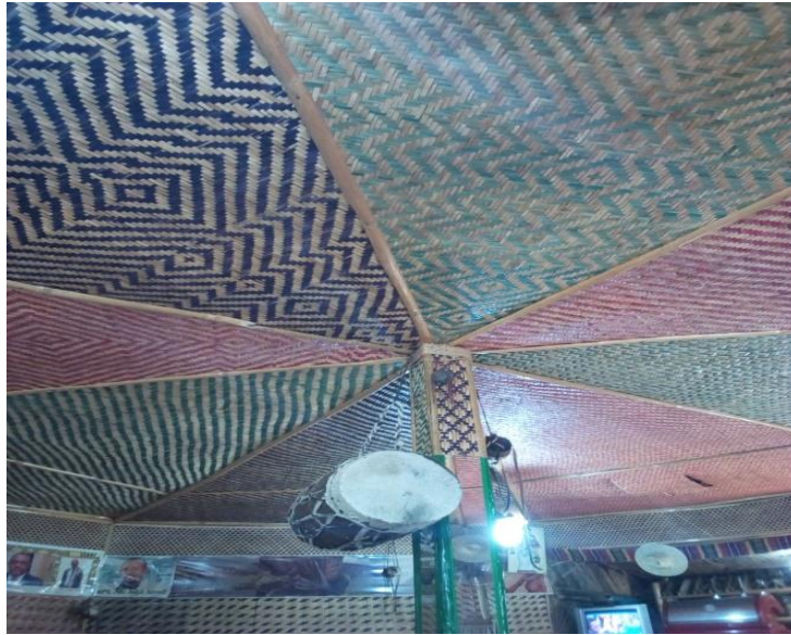
Figure 5: Improved bamboo ceiling (field observation)
