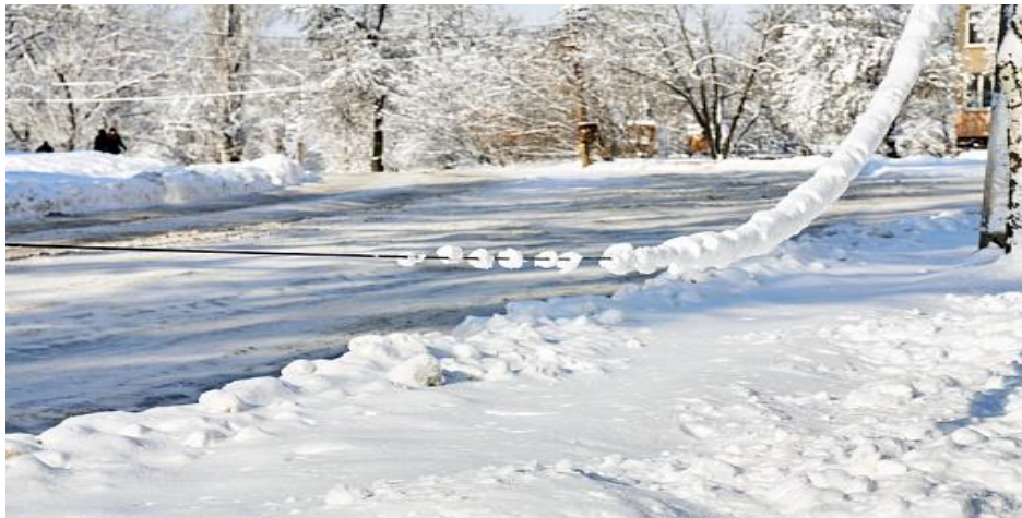
Figure 3.4. The effect of ice loading and wind force on OHTL
