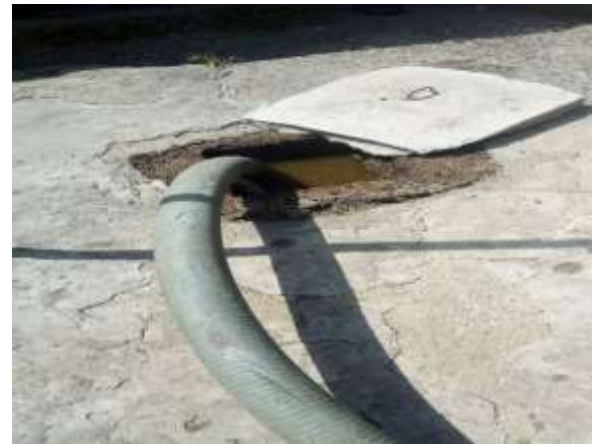
Figure 4.3b: Septic tank during emptying
