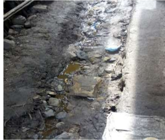
Figure 4.11b: Faecal sludge leakage from communal toilets
