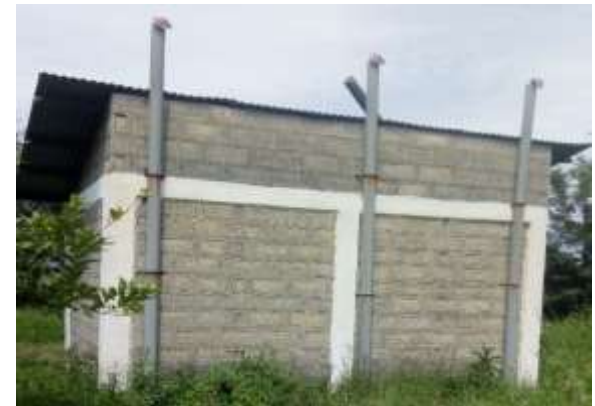
Figure 4.2 Vented Improved Pit (VIP) latrines
