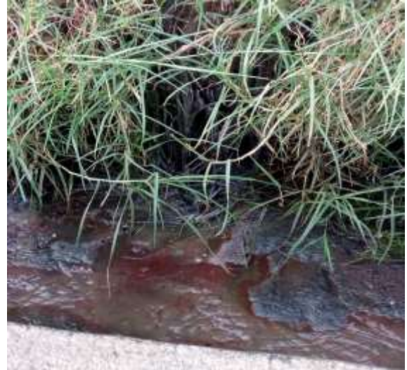
Figure 4.11a: Condominium septic tank overflow and discharged to open drain
