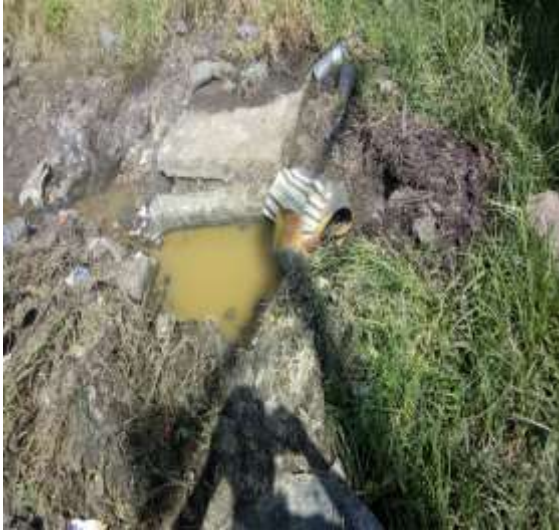
Figure 4.11a: Condominium septic tank overflow and discharged to open drain
