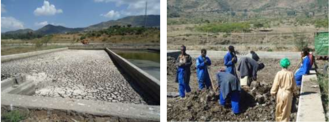
Figure 4.8: Cake/dried sludge removal from drying beds (photo by kedir 2009)
