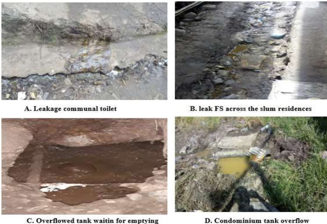
Figure 20: Pit latrine or septic tank leakage and overflows
