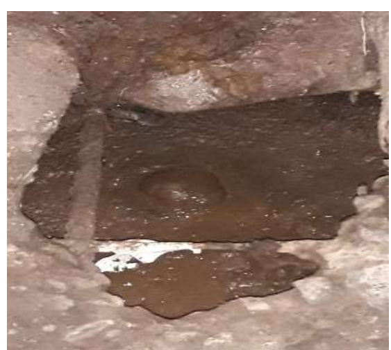
Figure 12e: Tank waiting for emptying
