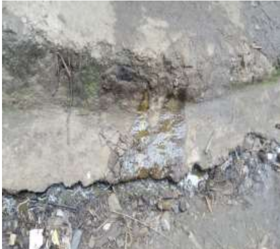
Figure 4.11b: Faecal sludge leakage from communal toilets
