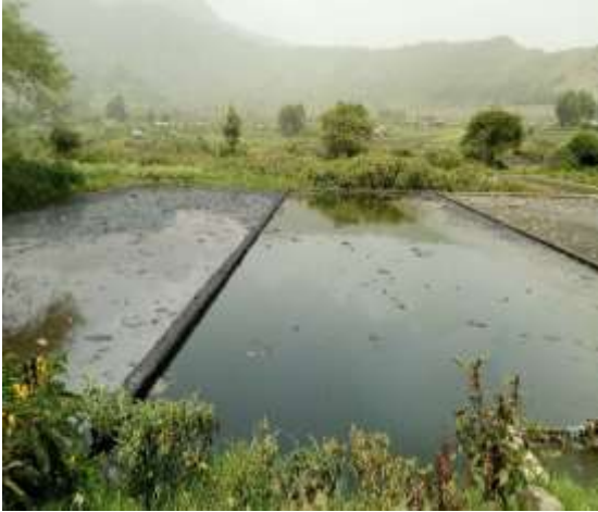
Figure 4.5a: Drying bed in use
