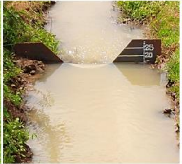
Graded V- Notch weir installed at QC
