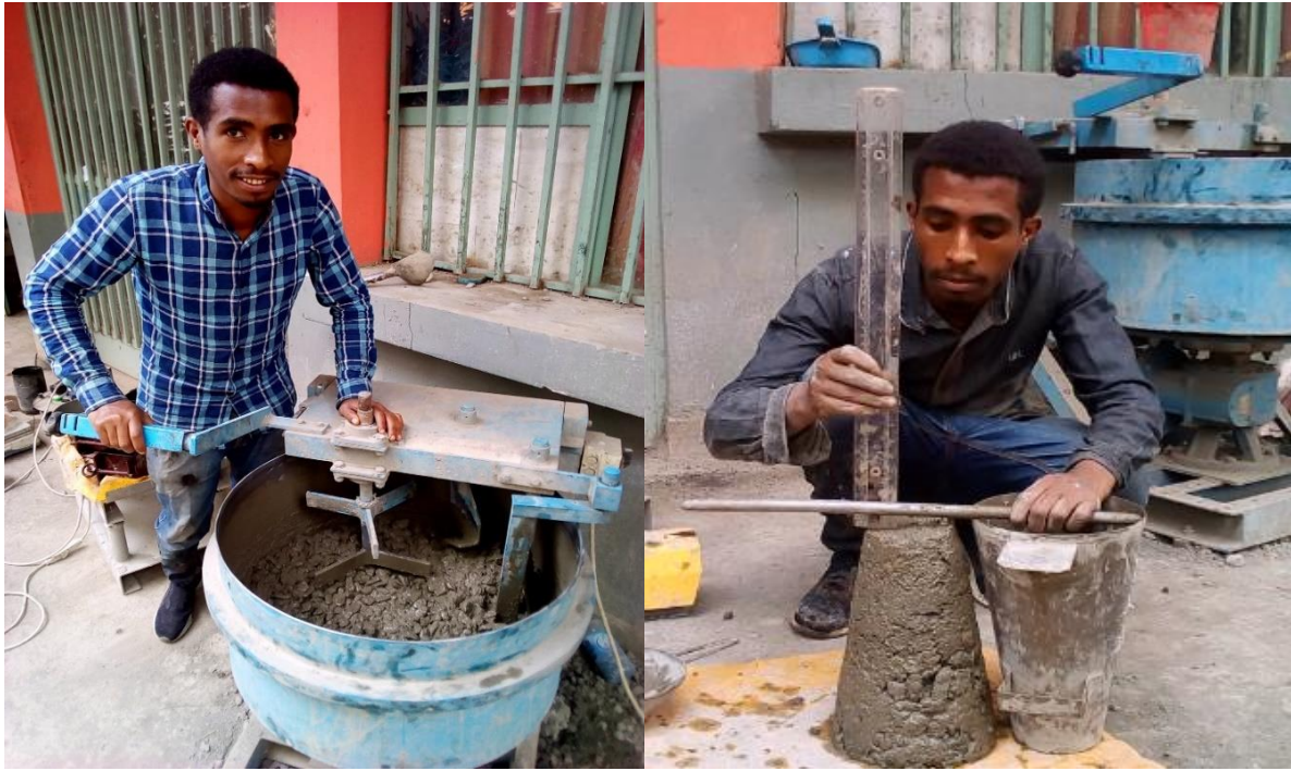
Figure 7-6: Concrete Mixing (left) and Slump Measurement (right)
