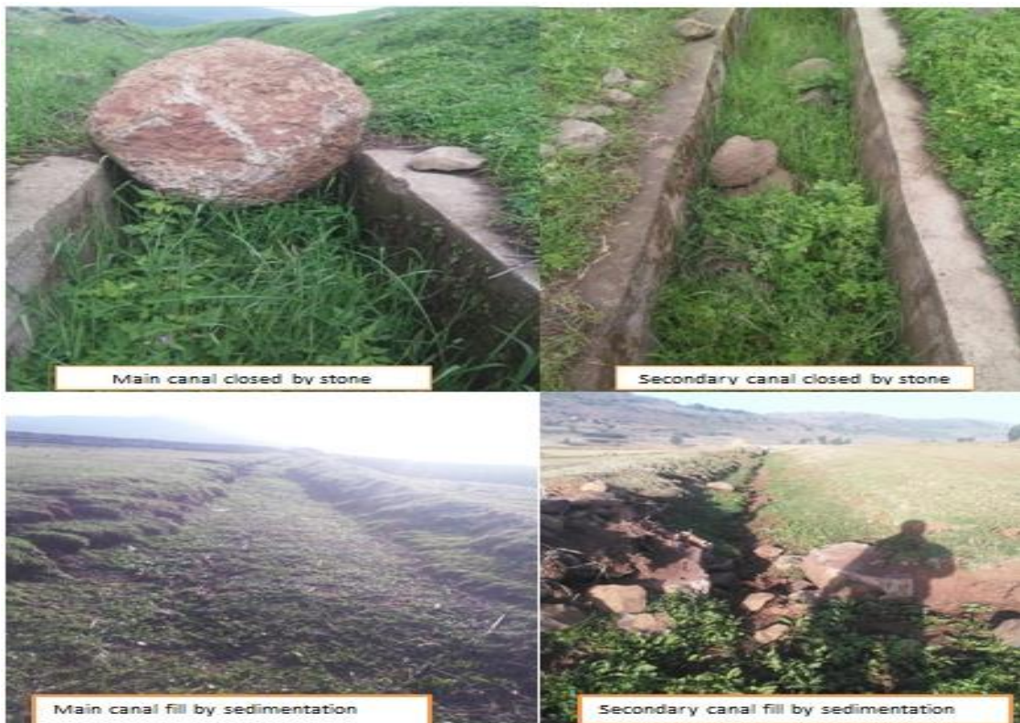
Appendix figure 3.3 Lined canal filled by sediment due to poor management of canal
