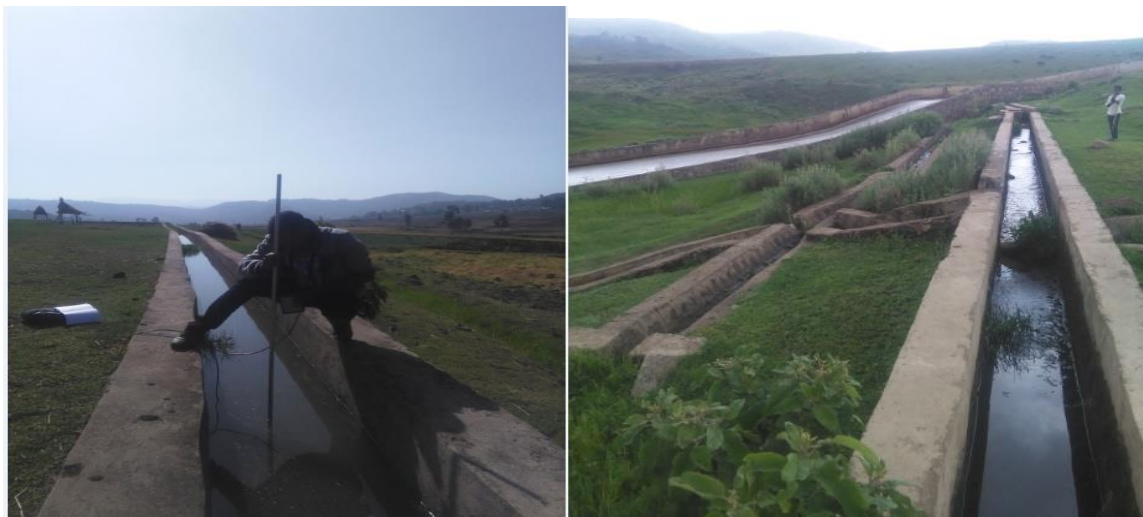
Appendix figure 3.7 Good condition Lined main and secondary canal
