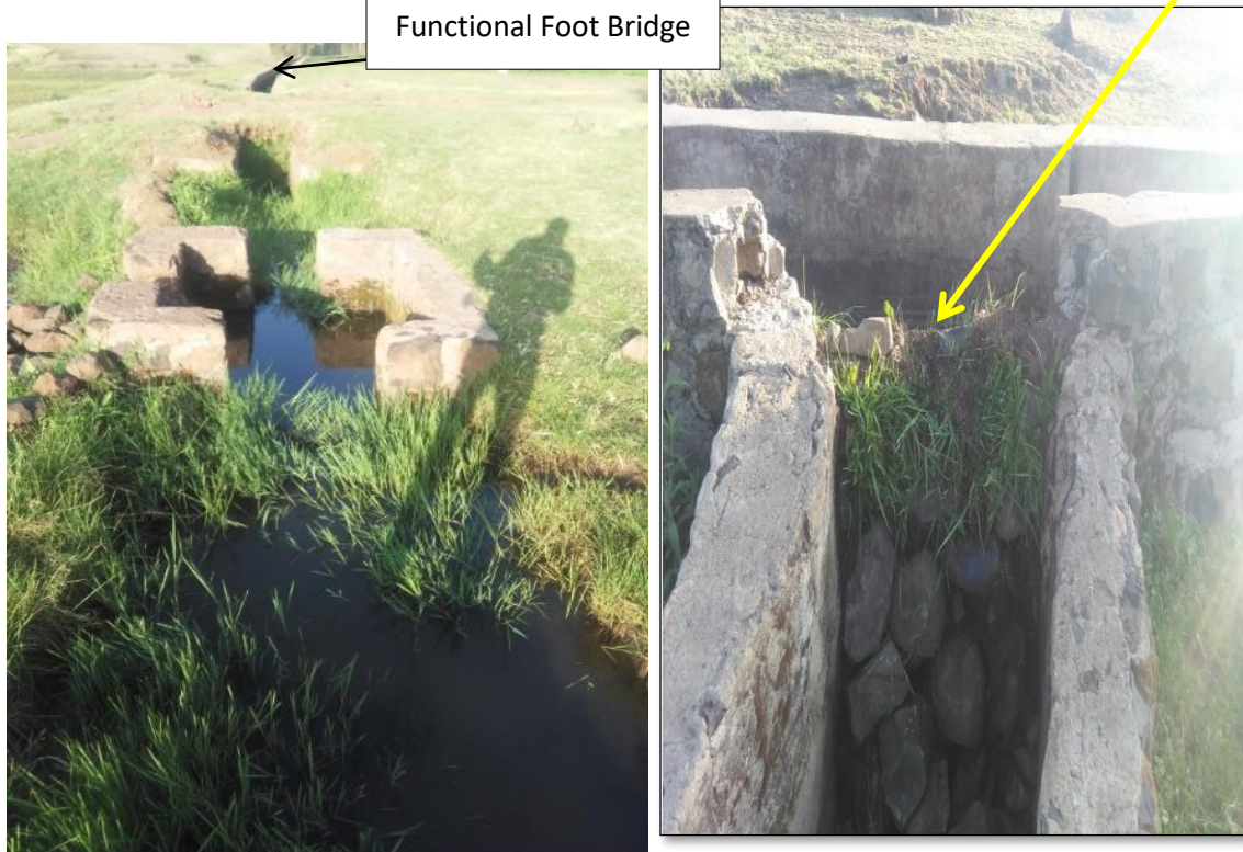
Appendix figure 3.3 Lined canal filled by sediment due to poor management of canal
