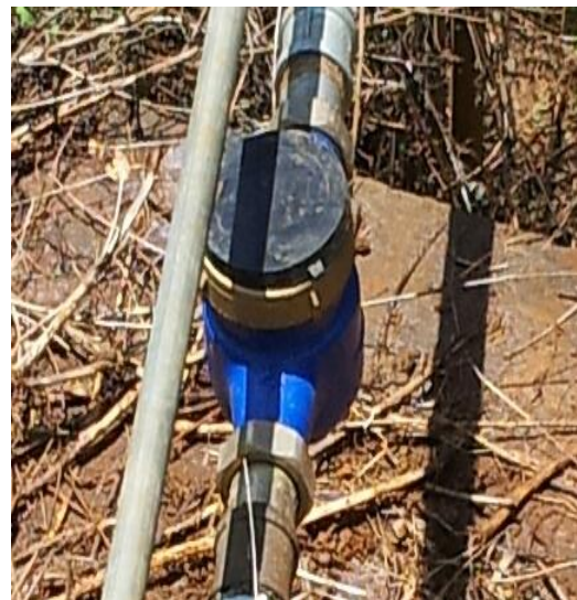
constructed water flow meter
