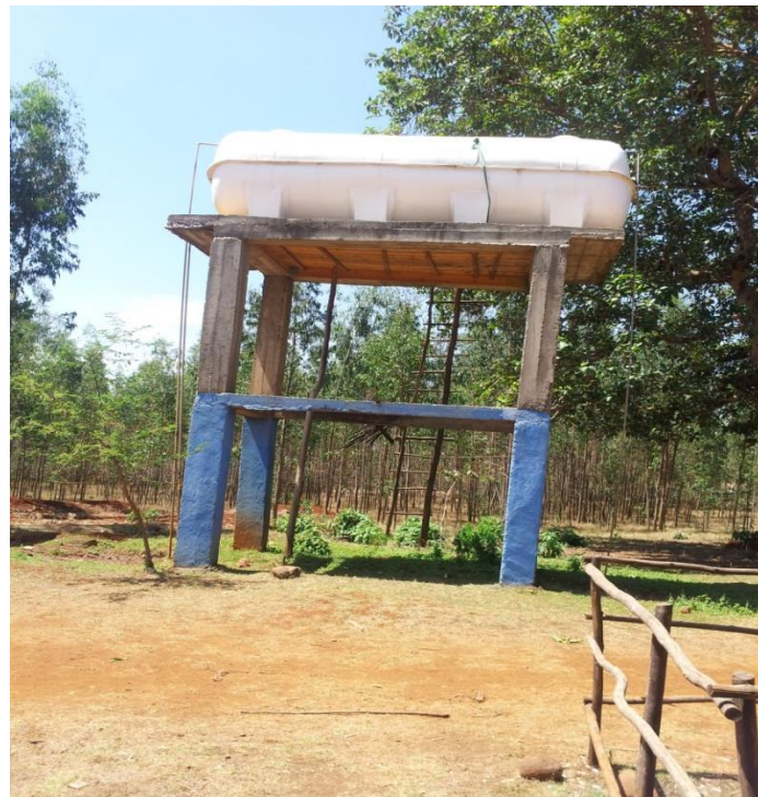
Figure 2.9: water storage tank
