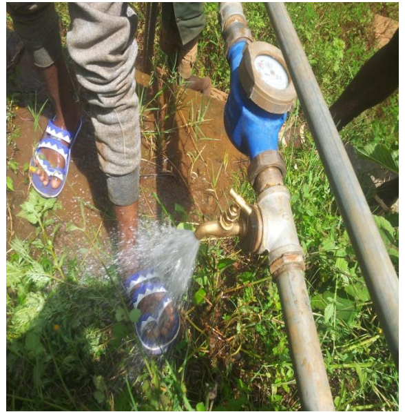
photo of gate valve after
