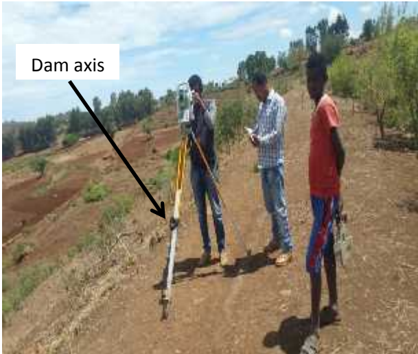
Field survey at the site
