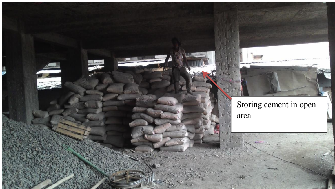
Figure 4.11: Common type of cement storing culture in Bahir Dar
