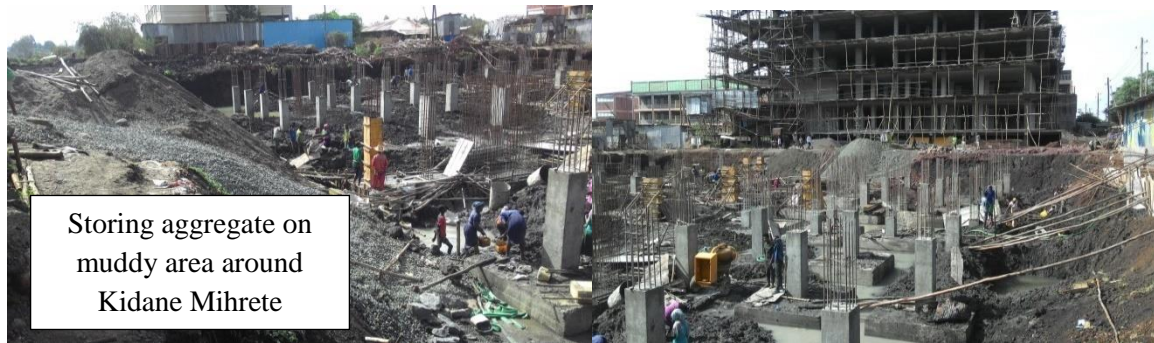
Figure 4.14: Photos taken from construction projects to show how aggregates are stored
